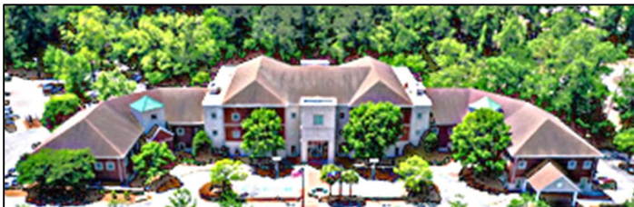
The Lexington Municipal Conference Center Building
